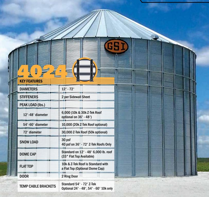
GSI stiffened bins use vertical stiffeners to channel the load of the bin to the foundation more effectively. The 4024 grain bin will match the corrugation of your other farm bins while adding storage capacity never seen before in a GSI 4" bin. If you have limited space available, the 4024 can be built up to 21 rings tall so you won't lose needed capacity with a smaller diameter. With the option of a 72' diameter, the 4024 is designed to expand as your operation grows.
